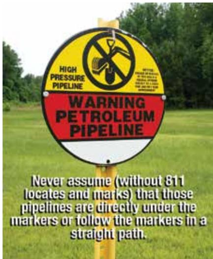
companies have pipelines on their land), gas transmission pipelines are also required to have pipeline markers at each crossing of a public road or railroad and wherever necessary to identify the location of the pipeline. Liquid pipeline regulations go a bit further in stating that those pipeline markers (in addition to at public road and rail crossing) shall be in sufficient number along the remainder of each buried line so that its location is accurately known.
